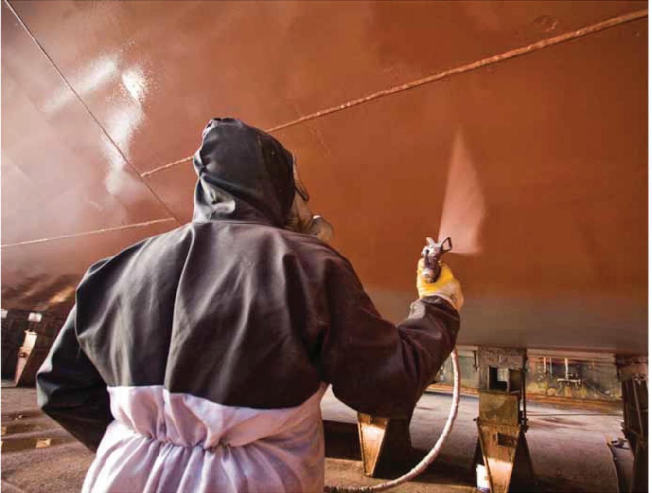
I-Tech is a company name that has become well-known in the marine paints and coatings industry in recent years. Its active agent Selektop®<sup>®</sup>, a substance which is added to antifouling coatings during the manufacturing process, repels barnacle larvae using a first-of-its-kind mode of action — it puts barnacle larvae looking to anchor themselves to a ship's hull into temporary swimming mode, rendering them unable to attach.
