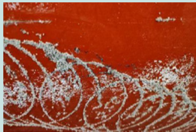
Vertical sides of a tanker coated with an FRC. Barnacles attached to mechanical damage areas. In service period: Unknown.
